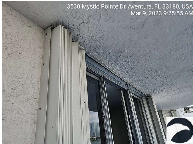
Photo 9. Shutters to be removed and reinstalled.
