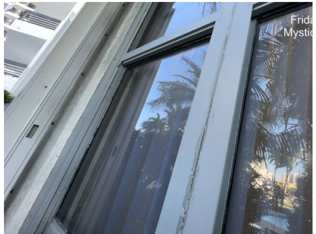
Photo 10. Windows to be painted.
