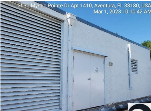
Photo 3. Roof structures and parapet wall to be painted
