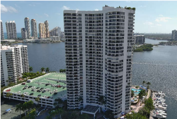
Photo 1. Building's exterior walls to be painted
