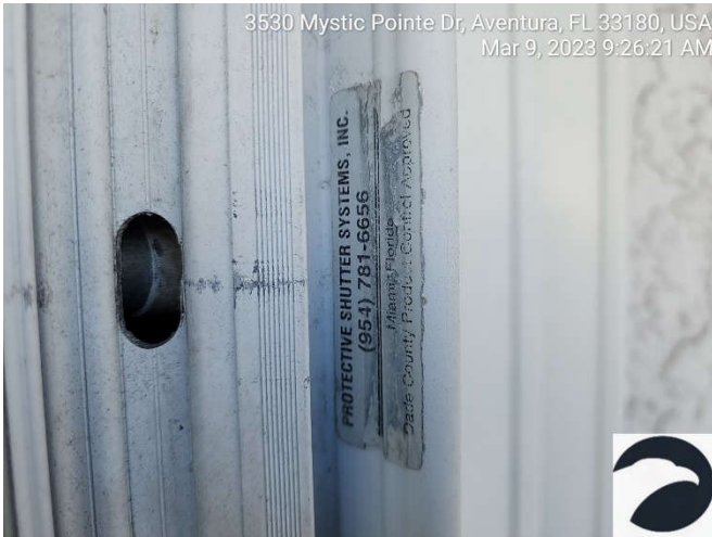
Photo 7.3.c.1 – Typical shutter system (Unit PH-8)
